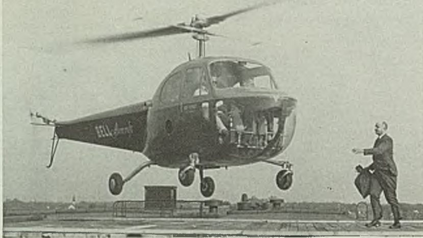
ROOFTOP LANDING: To demonstrate the practicability of helicopters landing on the roofs of buildings to pick up or deliver mail, this coupe-type craft lands on an improvised platform on the roof of Bell Aircraft Corp.'s Niagara Falls plant, where roof is stressed for 30 pounds per sq. ft. Holding the mail pouch is M. H. Ackerman, Post Office inspector-in-charge, directing helicopter mail projects
