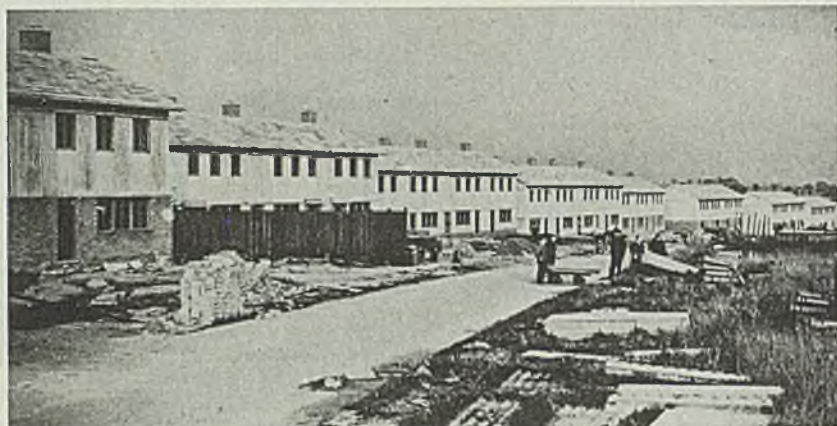
HOUSES FOR BRITAIN: These houses in Birmingham, England, have semi-steel, semibrick exteriors. To speed production, roofs are put on frameworks first so that construction can continue during inclement weather. About 800 of these will be ready for occupancy by Christmas. Acme photo
