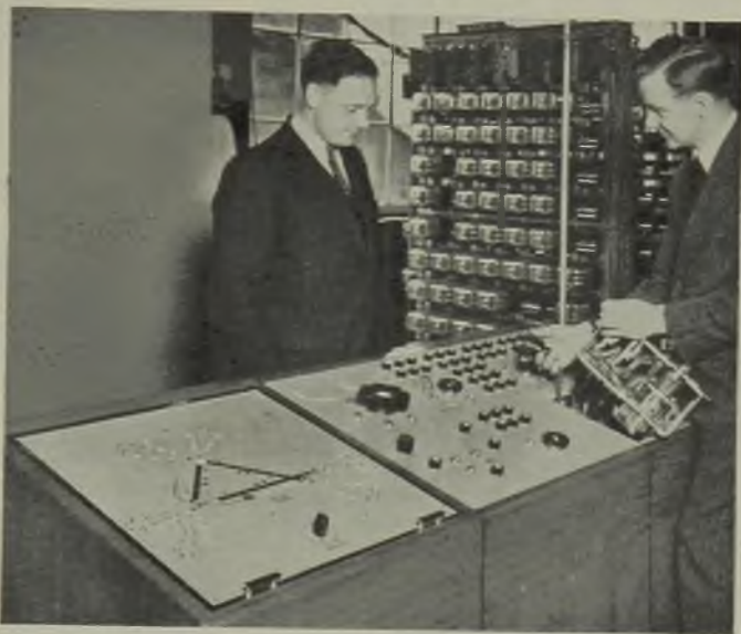
Lighting control desk with mimic airfield plan, showing lift-out panels for ease of maintenance and relay racks in background
