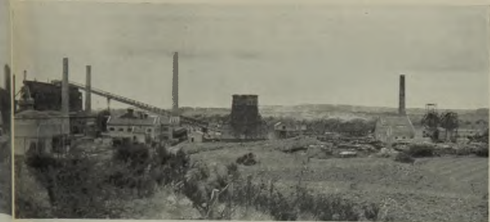
The Westwood Crude-Oil Works presents an impressive lay-out. Right to left: Pit from which the works receives part of its shale; cooling tower dealing with water from retort vapour condensers; ammonium sulphate plant; green shale conveyor to retorts; crude-oil storage tanks; oil and water scrubbers; products pump house; naphtha plant and storage; ammonia water storage; spent shale bings
