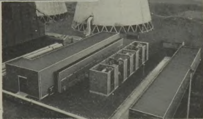
The new switch-house (left) runs parallel to the 6.6-kV switch-house right; interconnecting transformers between buildings
