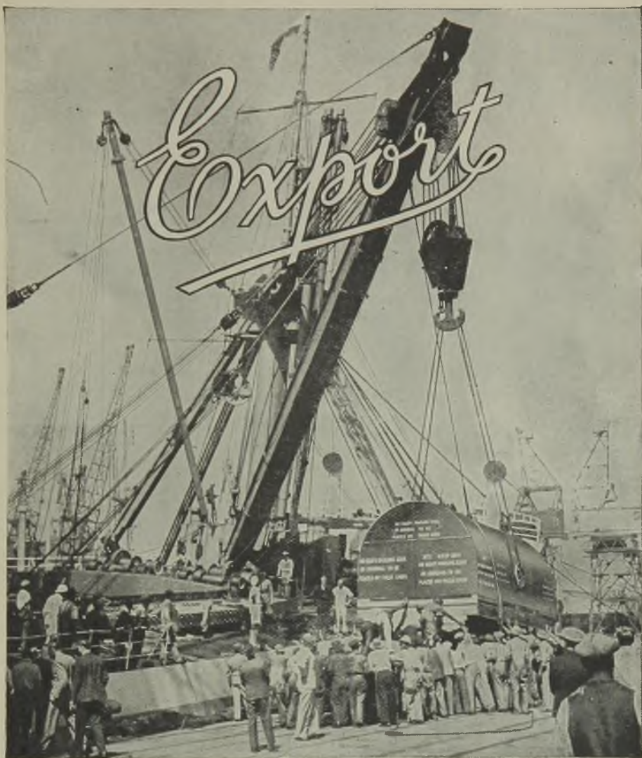
96-TON STATOR FOR A PARSONS 33,000-VOLT TURBO-ALTERNATOR BEING UNLOADED FROM THE FREIGHTER "CITY OF BARCELONA" AT TABLE BAY HARBOUR, SOUTH AFRICA
