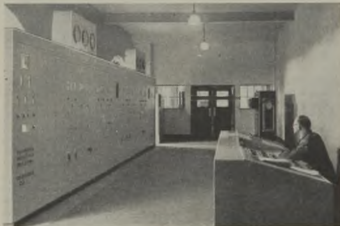
The main control board is in the power station
