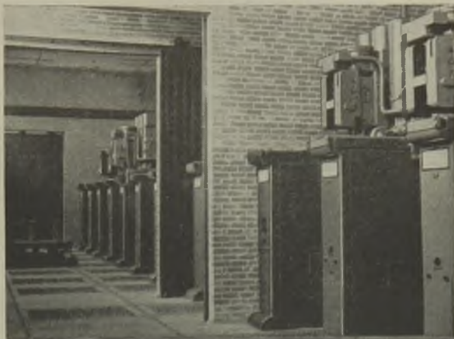
Between the two main switchrooms is the busbar section switch ; note rail track, truck, and fire-proof doors
