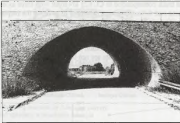
Fig. 11. View of the steel culvert in Poznań, Poland
