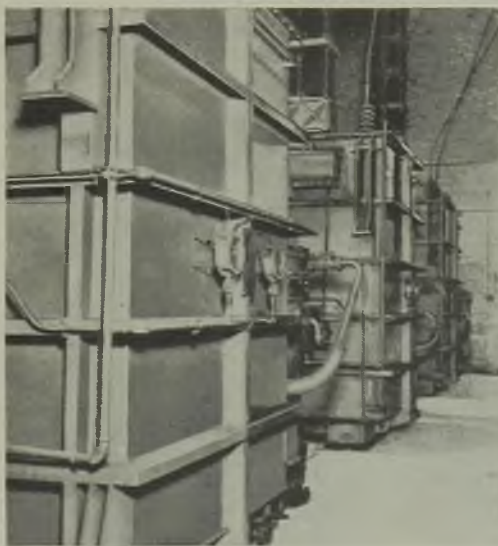
Above: From the 33-kV cables in each carbide-furnace transformer house, the circuit is led through two sets of hand-operated isolating switches and tubular busbars; note heavy l.v. busbars on left of picture. Each carbide-furnace transformer bank (left) consists of three single-phase 10,120-kVA transformers; normal working current is 46,000 A
