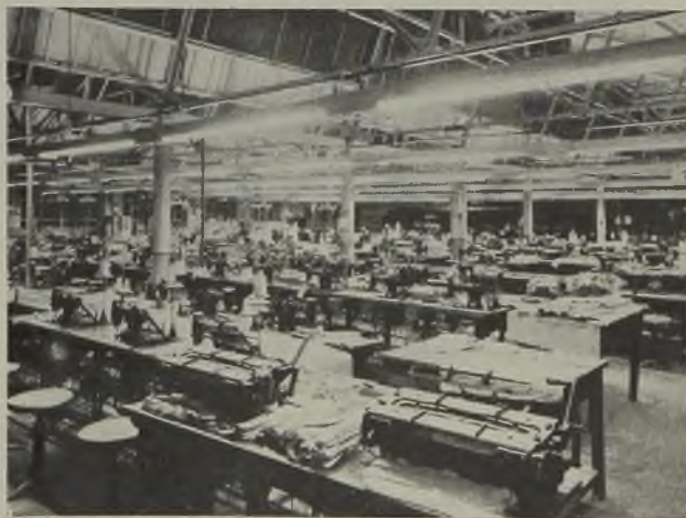
Guisborough Shirt Factory showing the new lighting installation
