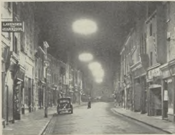
Experimental installation in High Street, Rugby
