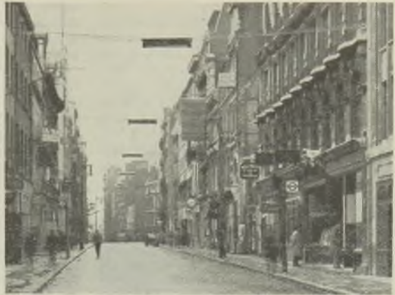
Daylight view showing special tubular fittings housing fluorescent lamps in Old Bond Street, London
