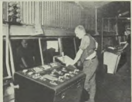
Rapid adjustment of the speed of the strip on the finishing stand is achieved by field control regulators, chain operated from the control pulpit
