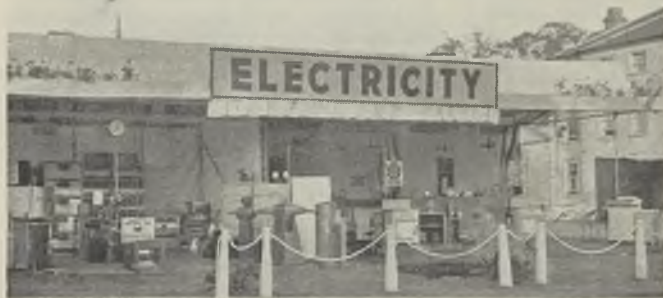
The joint exhibit of the Wolverhampton Electricity Department and the West Midlands J.E.A. at the Brewood Agricultural Show
