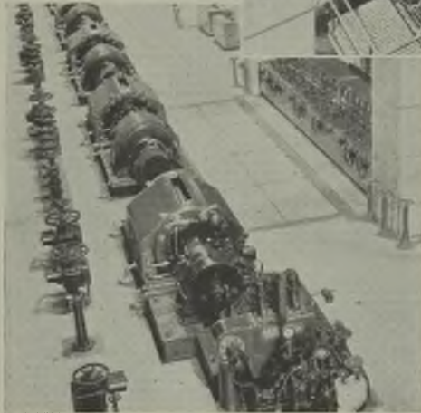
Above: Vertical 525-H.P. motor-driven pumps for circulating water. Left: Five feed pumps—four motor- and one steam-driven—in line in the western aisle or mechanical annexe
