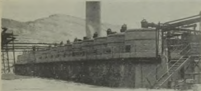
In the fractionating column the heated oil is "flashed" into its component parts; pipe-still in foreground and condensers and control room at rear. The heavy residue oil from the fractionating column is pumped into the coking stills (left)
