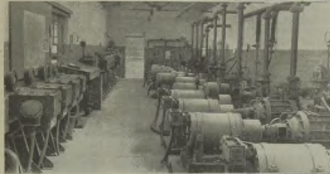
Line of fourteen units handling the motor spirit in final treatment stages. Large quantities of water are required, particularly for condensing; right, two 66-H.P. motor-driven sets in one of the pumping installations
