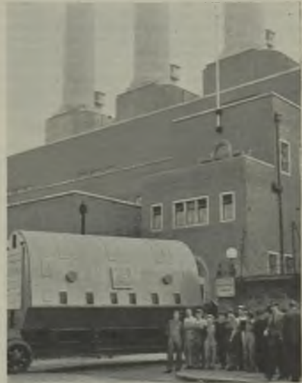
Arrival of the stator for the final turbine at Fulham power station
