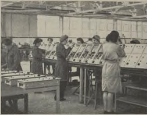
Assembling kitchen control units
