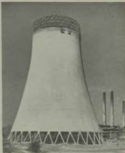
One of the pair of hyperbolic cooling towers nearing completion
