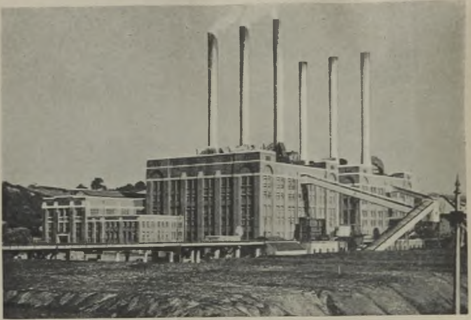
Electricity Generating Station built in Steel Frame Construction
