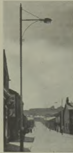
Metrovick "Trafford" lantern at Blackburn
