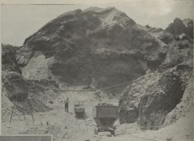
Spent shale is brought up out of an old bing by a single rope haulage system served by equipment with the motor incorporated in the rope drum (left)
