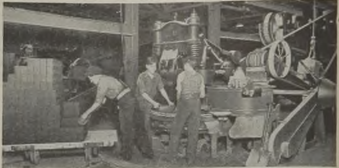
The moulding machine and the pan mill and associated conveyors constitute a production unit with a group drive
