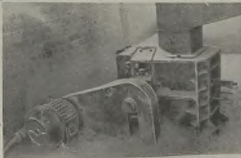
Lime is chute fed to a crusher
