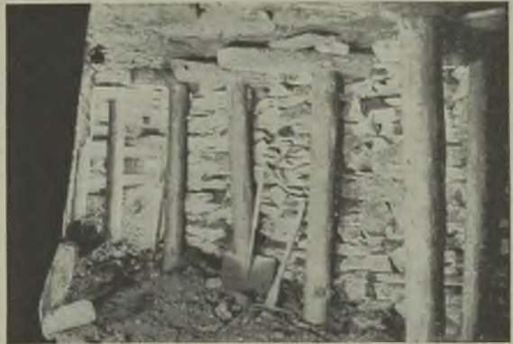
Goaf side of coal face showing the packs or walls which have to be built as the face advances
