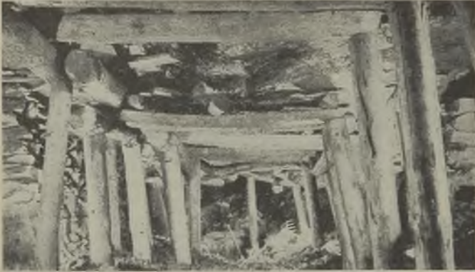
End of the road shown in the first illustration after coal has been removed
