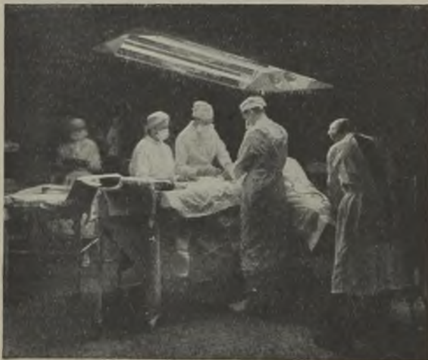
Fluorescent lighting in the operating theatre at Ancoats Hospital, Manchester
