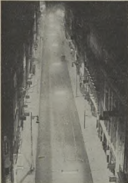
Old Bond Street installation using catenary-suspended "Warm-White" tubes
