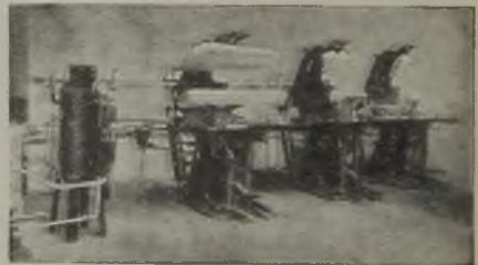
30 K.W. Boiler supplying steam for three pressing machines.
