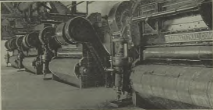
At Westwood four 30,000-lb per hr boilers (right), supply two 1,800-kW turbo-alternator sets (above)
