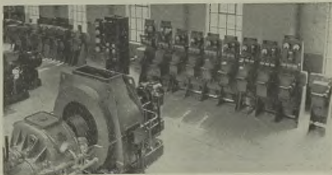
Between Addiewell and Westwood there is a direct 3.3-kV link; Addiewell h.v. switchgear (right) l.v. switchgear (left)
