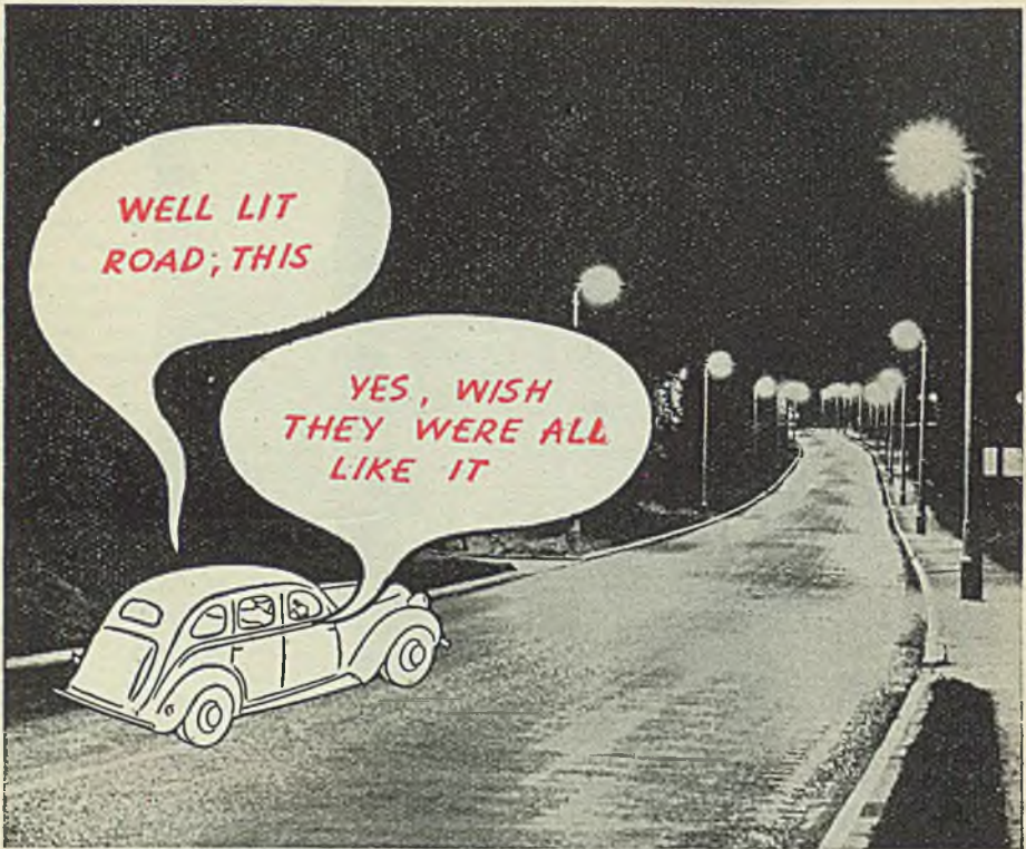
Engineering & Lighting Equipment Co. Ltd., "Golden Ray" Lanterns at 120' x 25' with Philips SO/H 140W Sodium Lamps.
