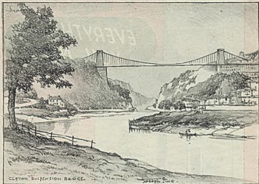
Bristol CLIFTON SUSPENSION BRIDGE Bridge 702 feet long from pier to pier. Spans the river Avon at a height of 245 feet. Completed 1864
