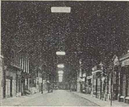
The B.T.H. centre-of-road scheme, seen from a Piccadilly balcony—8 500 lumens per 100 ft.
