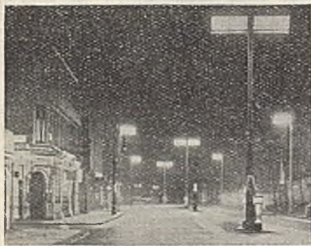
Night view of the Brompton Road installation giving 25 000 lumens per 100 ft. of road
