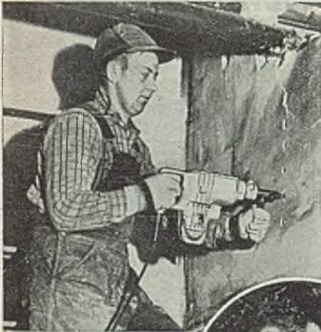
DEMOLITION IS QUICK and sure with the Thor-Nado portable electric hammer.
