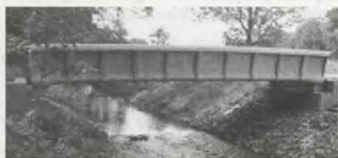
Fot. 9. Most z teksbetu w Oschatz [4] Pic. 9. The bridge with TRC
