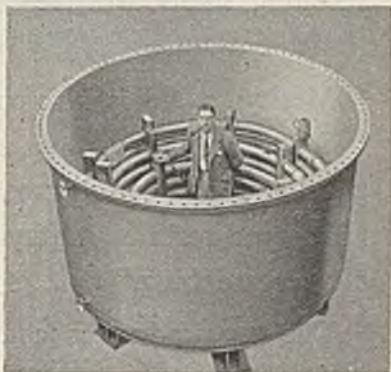
Homogeneous Lead Lined Vessel with three 3 in. Lead Coils
