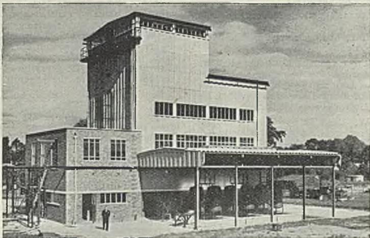
Pilot catalytic plant recently erected at Sunbury. The brick portion on the left houses the offices and laboratories connected with the pilot plant, which is in the tall part of the building. Its height is made necessary by the very tall reaction vessels used in the process.
