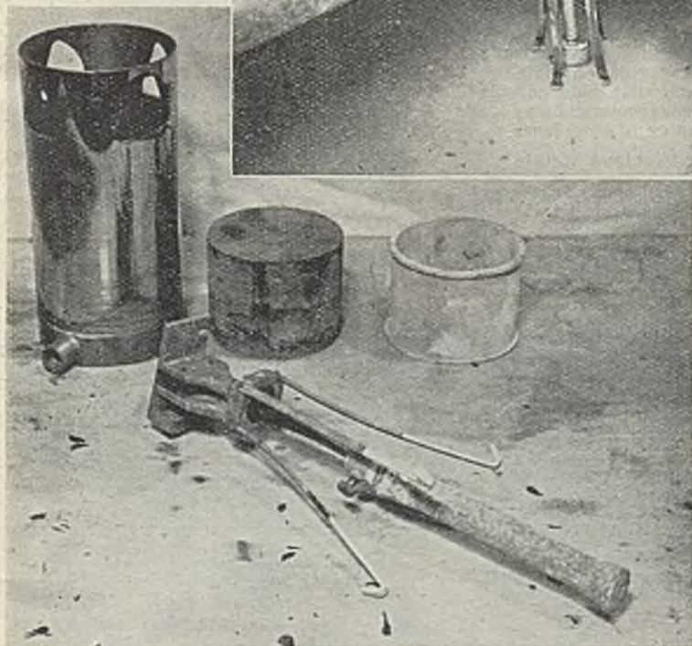
Fig. 6 (left). Cylinder liner showing registering block for registering rubber stopping-off sleeve, and also holding jig for central anode.
