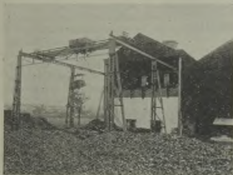
OVERHEAD ELECTRIC CRANE SERVING CUPOLA PLATFORM
