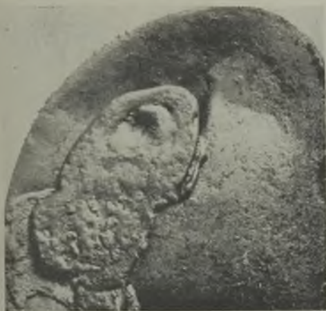
FIG. 16.—DEFECT CAUSED BY EXCESSIVE MOISTURE.
