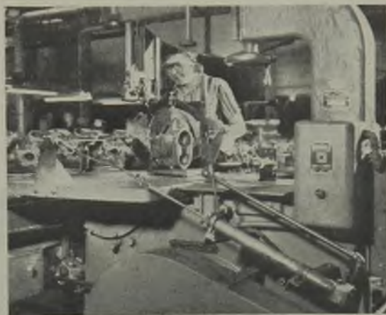
FIG. 15.—A BAND SAW IS USED FOR CUTTING OFF SPRUE.
