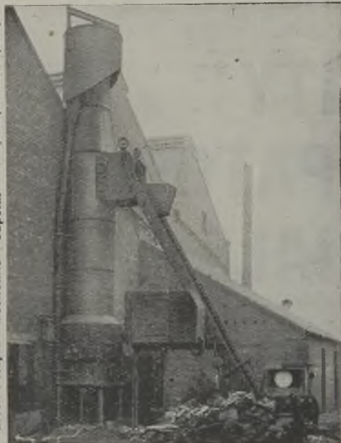
Green's Rapid "Economic" Cupola. 1 to 20 tons per hour capacity.
