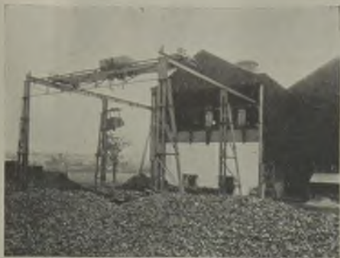
OVERHEAD ELECTRIC CRANE SERVING CUPOLA PLATFORM
