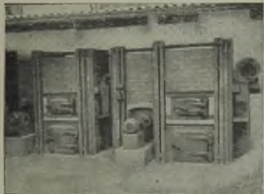
2 Brick built for large Stoves
