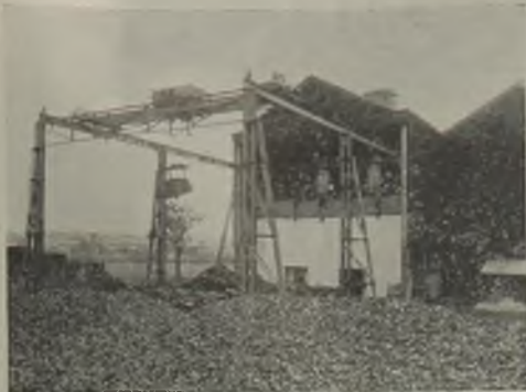
OVERHEAD ELECTRIC CRANE SERVING CUPOLA PLATFORM
