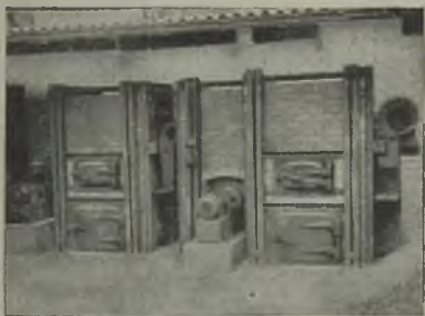
2 Brick built for large Stoves
