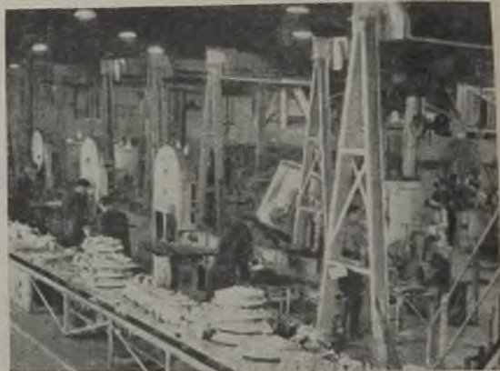
FIG. 25.—GENERAL VIEW FROM NORTH-EAST CORNER.
