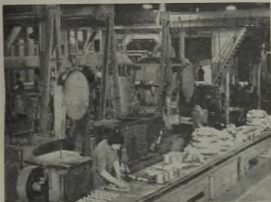
FIG. 26.—GENERAL VIEW OF SOUTH-EAST CORNER.
