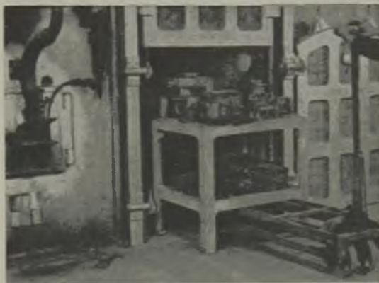
FIG. 31.—DIE-RACK LOADED WITH DIES BEING PLACED IN HEATING CHAMBER.
