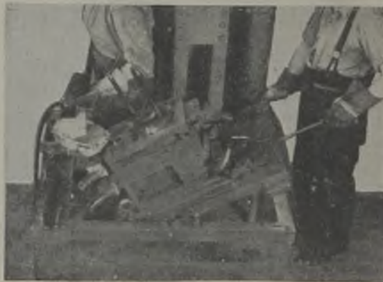
FIG. 15.—POURING COOLANT INLET CASTING.
