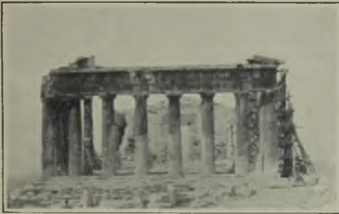
THE PARTHENON ON THE ACROPOLIS BUILT OF MARBLE OR MASSIVE LIMESTONE FROM THE QUARRIES OF MOUNT PENTELICUS.
