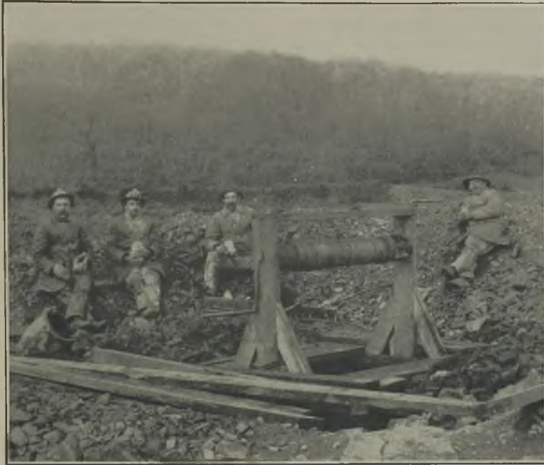
TREFUSIS SHAFT IN THE WHEEL UNITY WOOD SECTION, WHICH GIVES ACCESS TO A BRANCH OF THE ADIT WHICH DRAINS THE LODES SOUTH OF AND INCLUDING THE MIDDLE LODE TO A DEPTH OF APPROXIMATELY 36 FATHOMS FROM SURFACE, ACCORDING TO THE CONFIGURATION OF THE COUNTRY.
