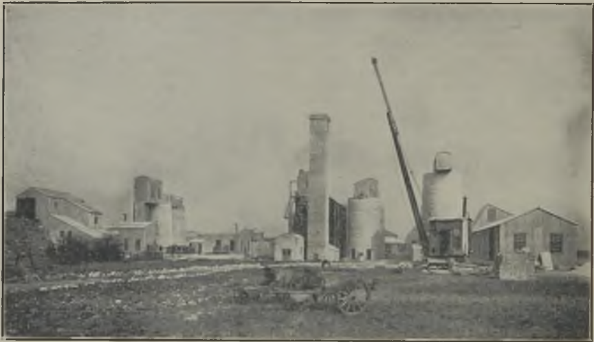
GENERAL VIEW OF BARNSTONE CEMENT WORKS.
