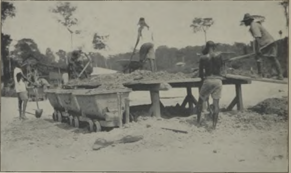
FIG. 8.—LOADING PLATFORM FOR TRUCK HAULAGE.
