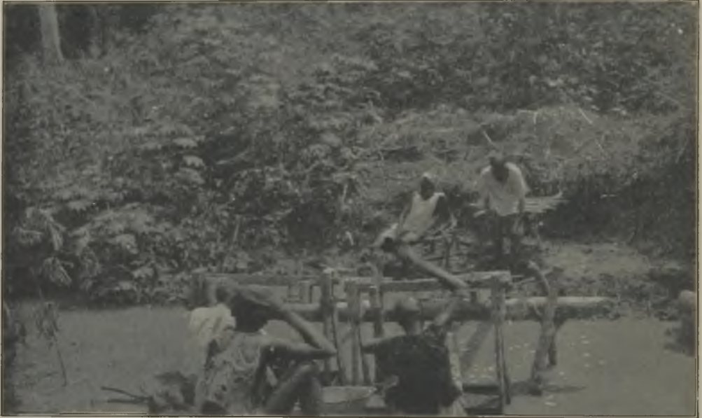
FIG. 6.—JOPLIN JIG AT WORK.
