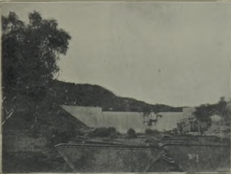
FIG. 4.—RIFLE CREEK DAM FROM BELOW.
