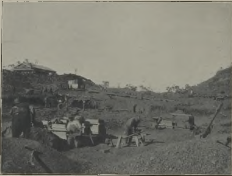
FIG. 5.—EXCAVATIONS FOR THE LOWER MILL.
