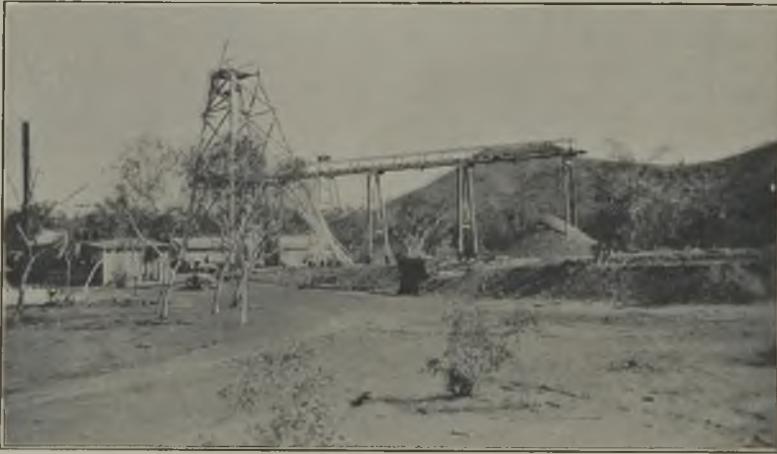
FIG. 3.—HEADFRAME AT LAWLOR SHAFT.
