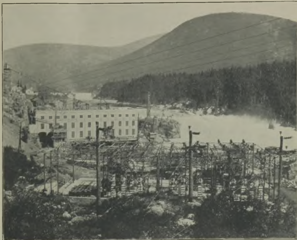
HYDRO-ELECTRIC STATION AT LOWER BONNINGTON FALLS.
