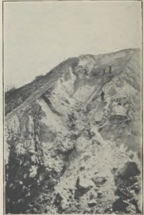
FIG. 3.—BAKAU MAIN FACE—BARRING DOWN WEATHERED TOPAZ-APLITE.
