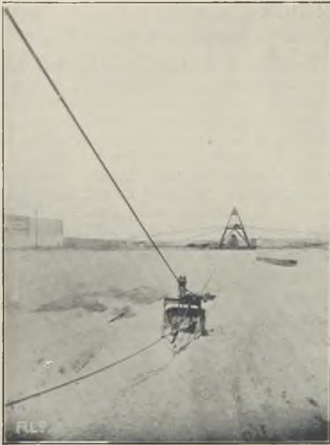
FIG. 2.—BUCKET OF DRAGLINE EXCAVATOR DIGGING.
