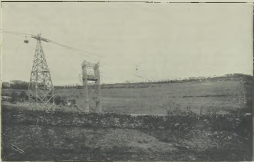
FIG. 8.—LONG SPAN ON ROPEWAY IN FRANCE.
