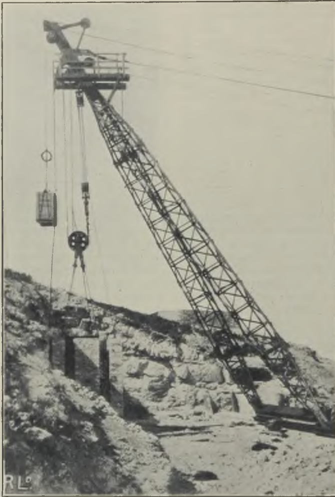
FIG. 6.—TAIL MAST OF RADIAL CABLEWAY OPERATING IN IRON-ORE QUARRY IN SPAIN.
