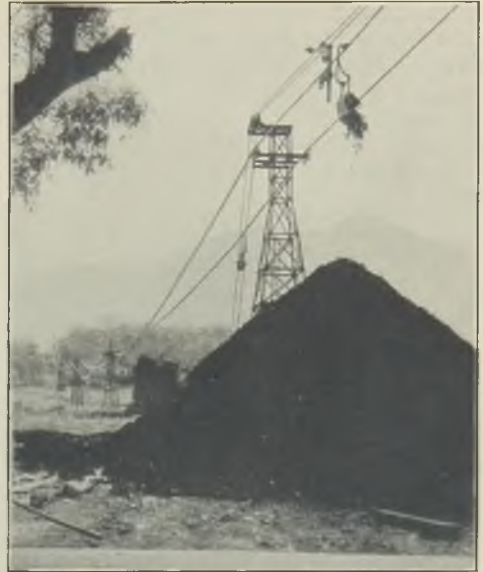
FIG. 4.—BUCKET TIPPING ON ROPEWAY IN INDIA.
