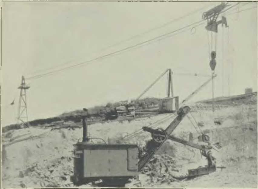
FIG. 5.—ROPEWAY WORKING IN CONJUNCTION WITH STEAM SHOVEL.
