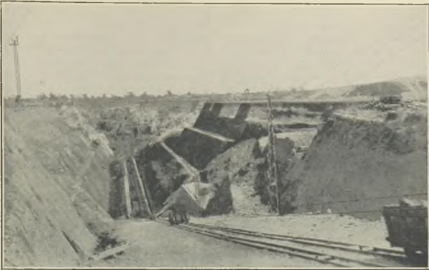
FIG. 4.—RUASHI OPEN-CAST—FACING EAST.
