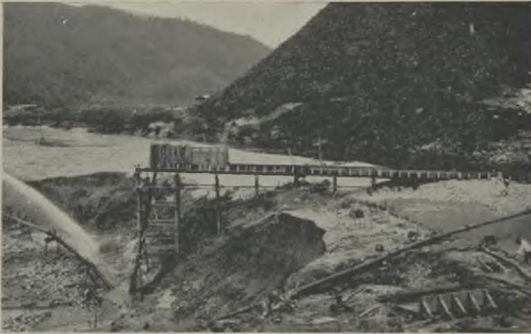
HYDRAULIC ELEVATOR AT WORK ON NARE RIVER.
