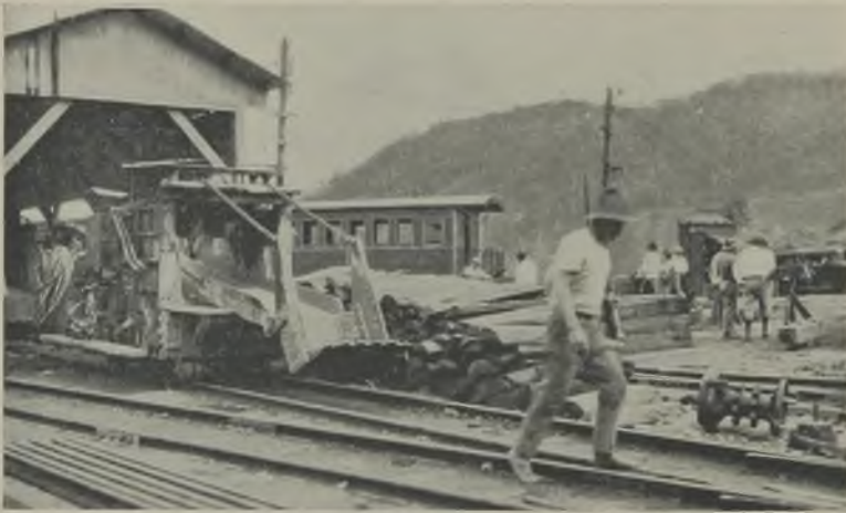
POWER-SHOVEL USED IN TUNNEL ON RAILWAY BETWEEN MEDELLIN AND THE MAGDALENA RIVER.
