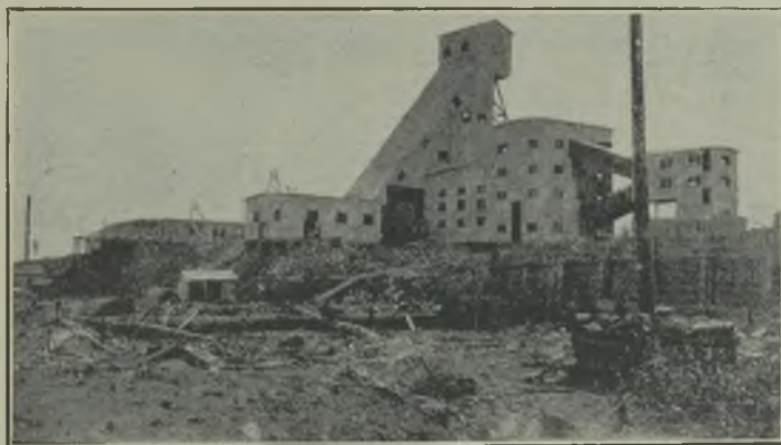
HEADFRAME AND CRUSHER HOUSE, NO. 3 SHAFT.
