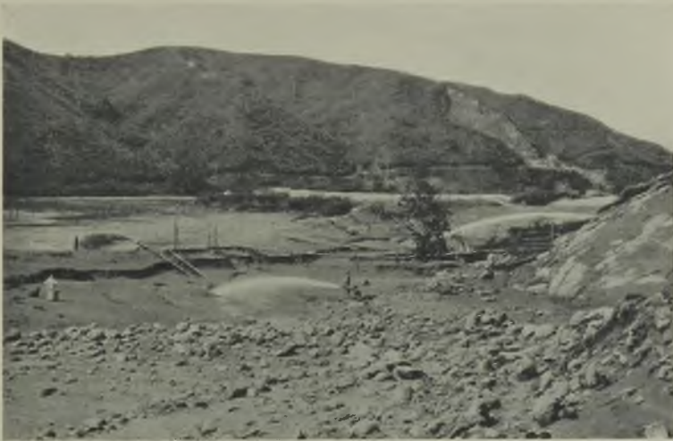
STARTING A HOLE ON THE PORCE RIVER.
