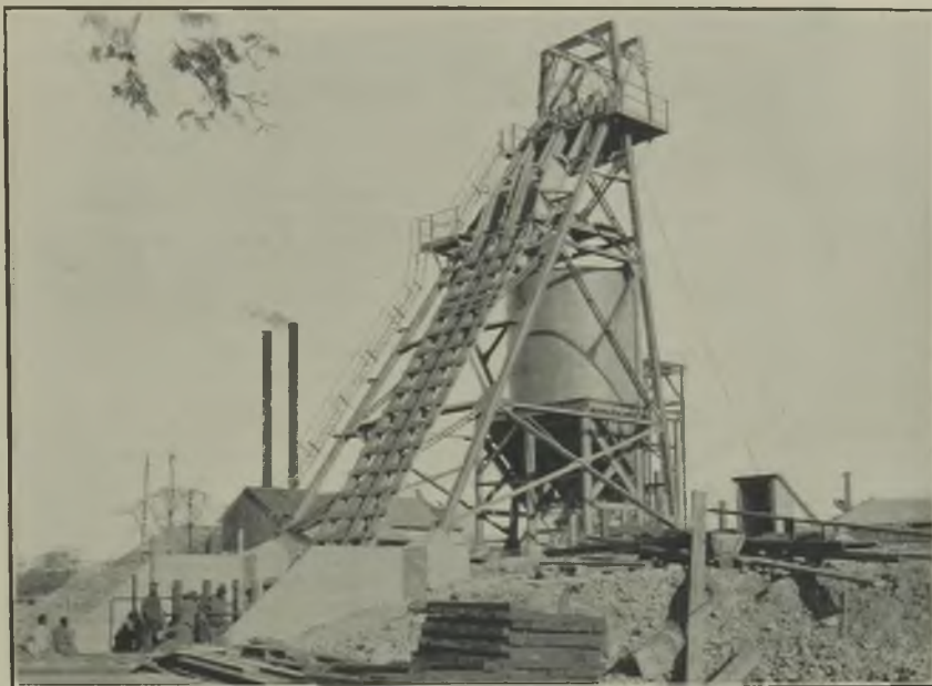
FIG. 2.—DEVELOPMENT STEEL HEADFRAME AT NO. 2 SHAFT.
