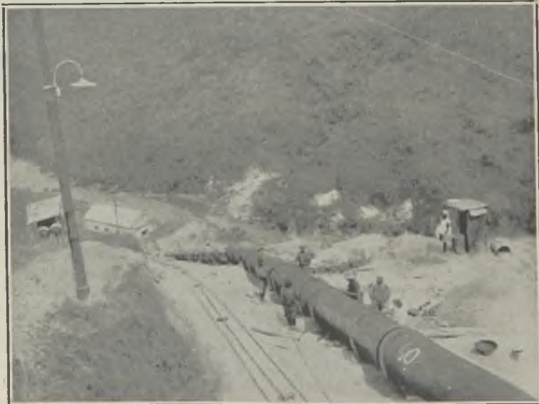
LOWER END OF PIPE LINE.
