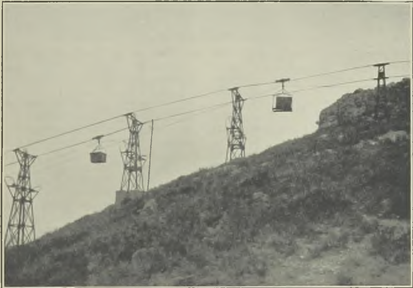
FIG. 4.—SPACING OF TRESTLES OVER CONVEX PROFILE.
