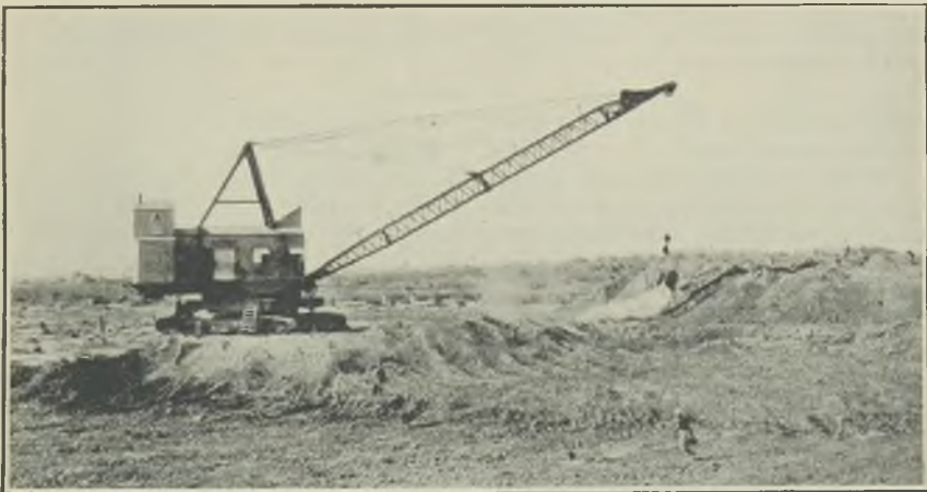
FIG. 1.—DRAGLINE AT WORK ON THE SUKKUR BARRAGE.
