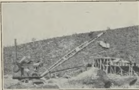
FIG. 6.—DRAGLINE WORKING AURIFEROUS GRAVEL IN ALASKA.
