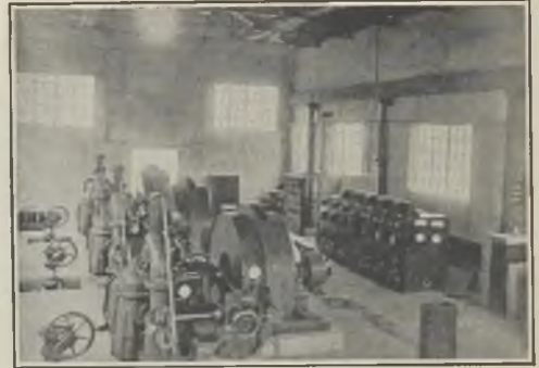
INTERIOR OF POWER HOUSE.
