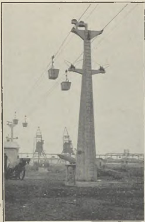
FIG. 2.—REINFORCED CONCRETE TRESTLE.
