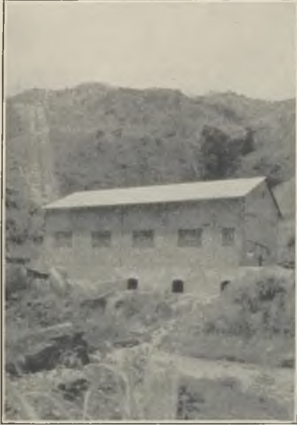
POWER HOUSE AND PIPE LINE.
