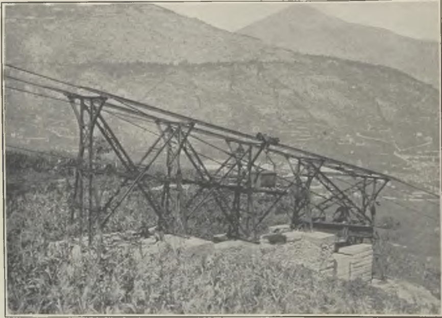
FIG. 5.—INTERMEDIATE ANCHORAGE AND STRETCHING GEAR.
