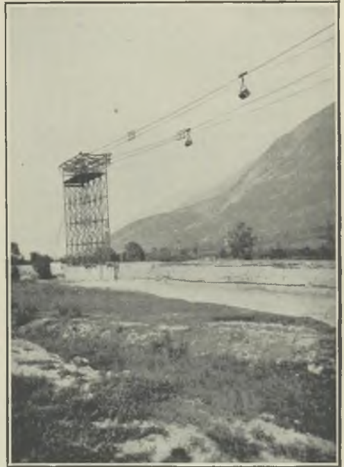
FIG. 1.—ROPEWAY STATION, SHOWING HAULING AND CARRYING ROPES.
