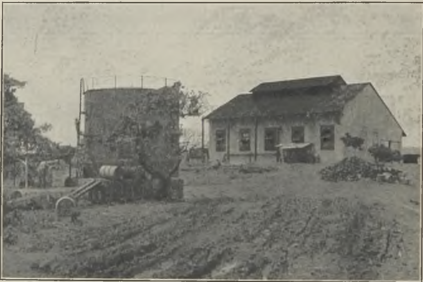
ELECTRIC POWER-HOUSE AT CALAMACITO FOR THE REMANCE MINE.
