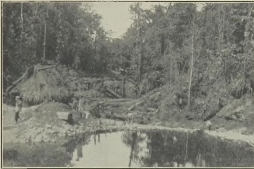
PENSTOCK DAM FOR THE EL MINERAL PIPE-LINE.
