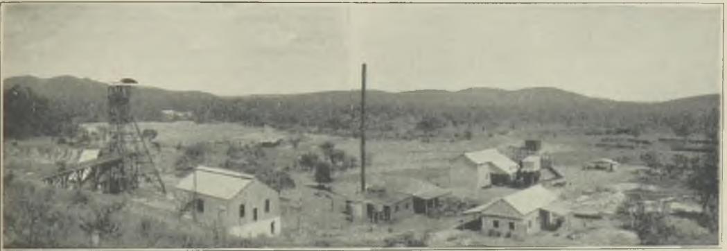
GENERAL VIEW OF THE ABENAB MINE: OPEN-CAST ON THE EXTREME LEFT.
