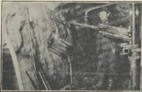
SET-UP FOR DEEPCOLE DRILLING.
