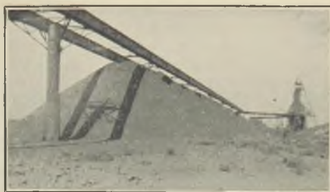
FIG. 2.—STEEL TOWER FILLED WITH CONCRETE IN STOCK-PILE CARRYING ABOUT 2,000 TONS OF ORE PER LINEAL FOOT OF TRESTLE.
