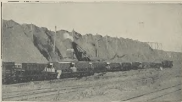
FIG. 1.—STEAM SHOVEL LOADING ORE FROM STOCK-PILE: MAAS MINE, CLEVELAND CLIFFS IRON CO.
