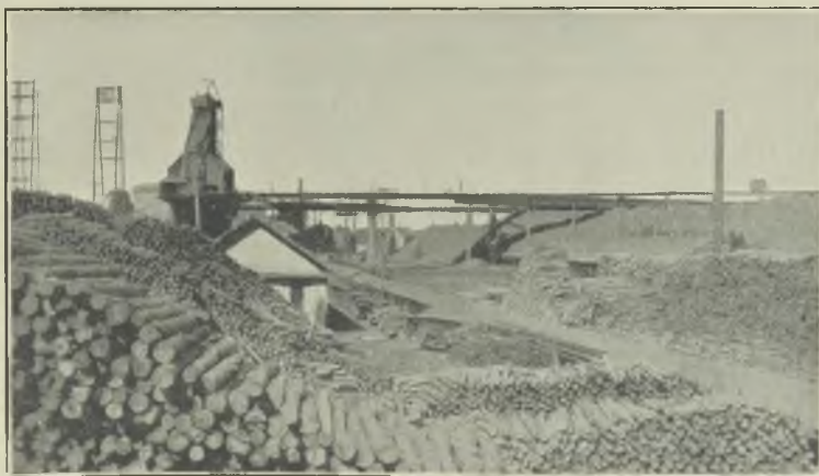
FIG. 3.—MINE TIMBER AND COVERED TRACK TO SHAFT: ATHENS MINE, CLEVELAND CLIFFS IRON CO.
