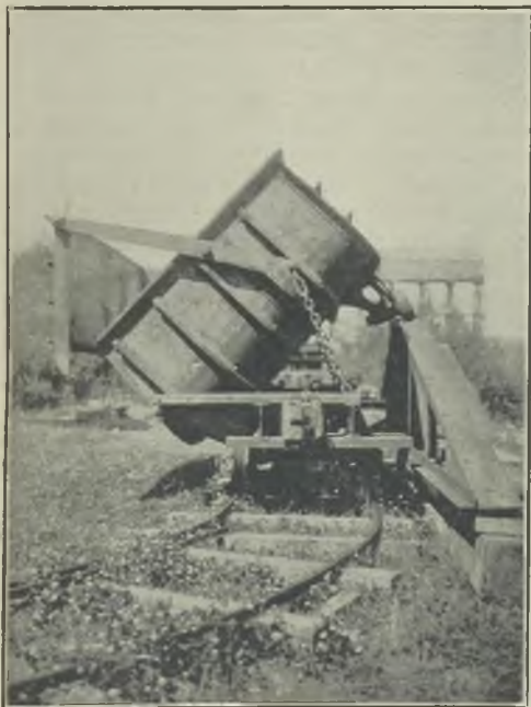
FIG. 2.—GRANBY 3 FT. GAUGE MINE CAR WITH 45° DUMPING ANGLE.
