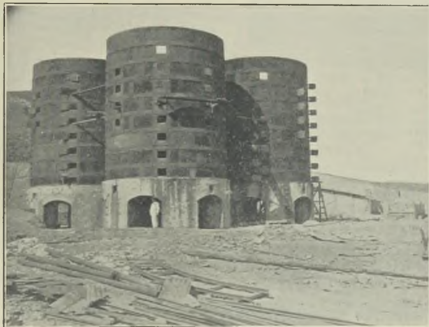
FIG. 1.—FURNACE SHELLS AND BASEMENTS FOR DRIVING GEAR.
