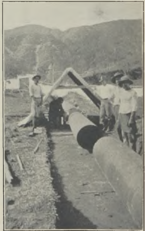
FIG. 7.—No. 2 WELDER JOINING PIPES.
