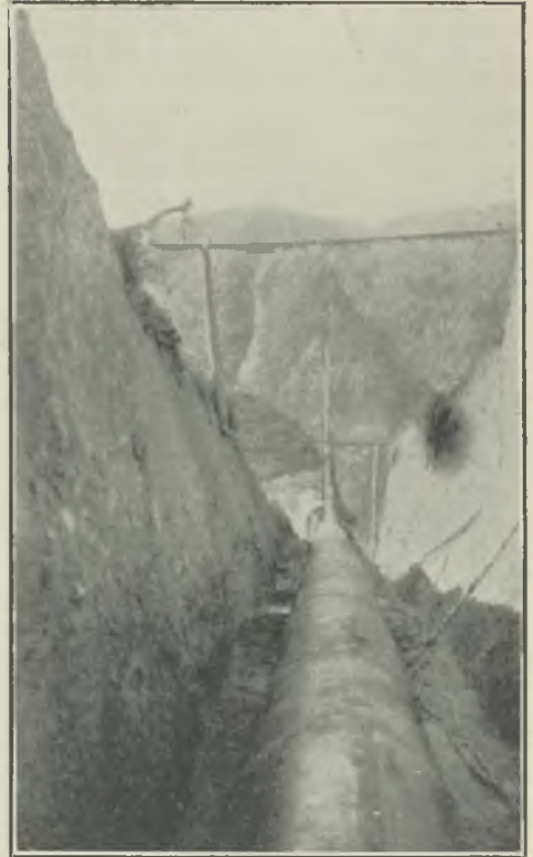
FIG. 9.—PIPELINE LEAVING INTAKE AND EMERGING FROM INCLINED RISE.
