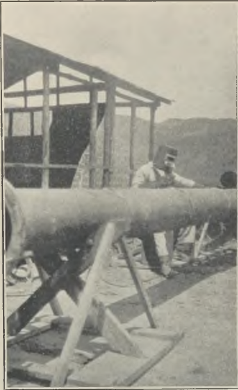
FIG. 6.—No. 1 WELDER, HAVING TACK-WELDED SINGLE 4 FT. PIPES TOGETHER, COMMENCES CIRCUMFERENTIAL WELDING.
