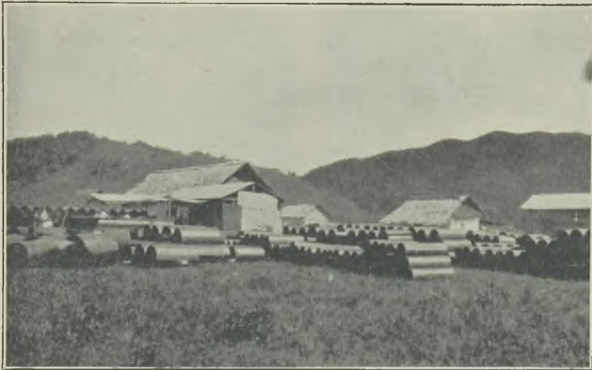
FIG. 5.—ROLLED PIPESHEETS AWAITING WELDING.
