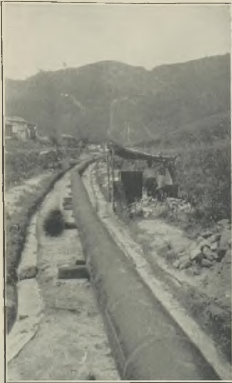
FIG. 8.—WELDING MACHINE ALONGSIDE PIPELINE.
