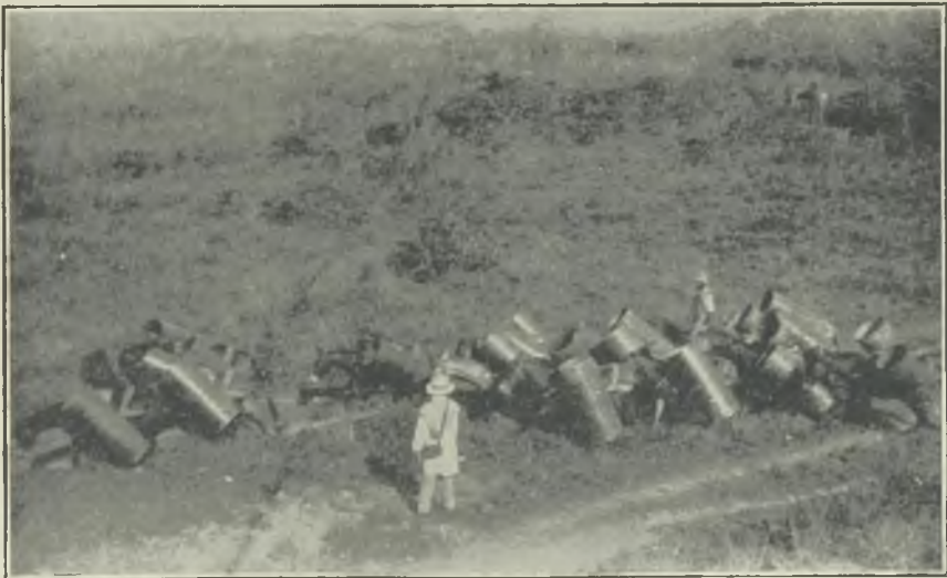
FIG. 3.—MULE TRANSPORT OF 26 IN. PIPES.
