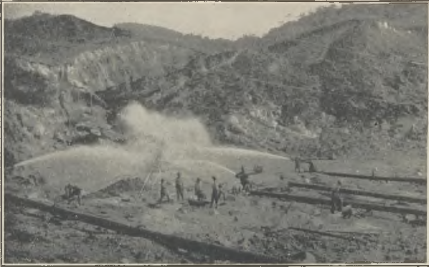
FIG. 10.—PART OF THE WORKING PADDOCK—12 IN. LINES.
