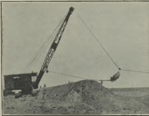
FIG. 4.—SCRAPER LIFTED CLEAR OF WORK AND RETURNING TO PIT BY GRAVITY.
