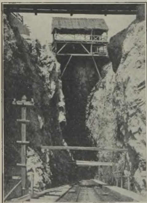
FIG. 4.—HAULAGE INCLINE PASSING INTO TUNNEL AT BEATRICE MINE.
