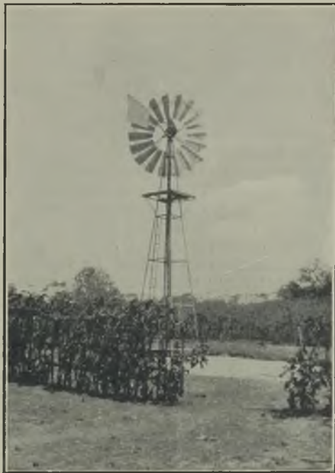
FIG. 18.—THE FIRST DRILLED WELL AND WIND-MILL PUMP IN UGANDA, AT KATAKWE, EASTERN PROVINCE.
