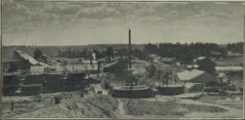
GENERAL VIEW OF REDUCTION WORKS, SUB NIGEL MINE.
