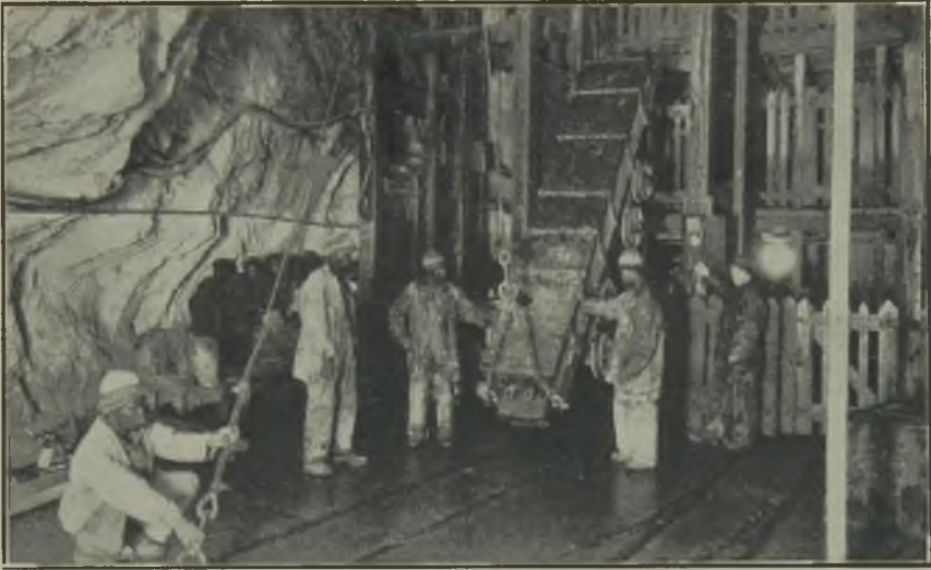
SUB NIGEL MINE—UNLOADING DRILL CONTAINER UNDERGROUND.
