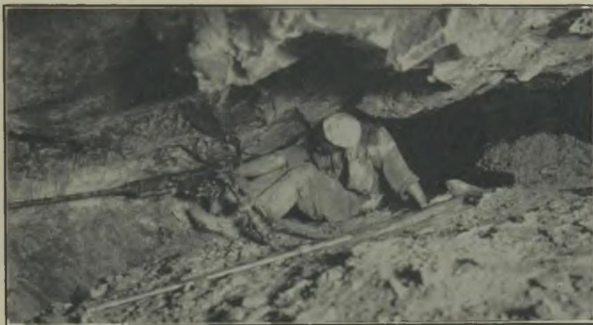
SUB NIGEL MINE—NATIVE DRILLING, WITH SCRAPER IN OPERATION IN BACKGROUND.
