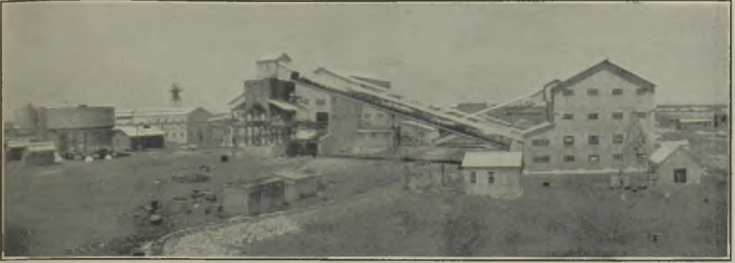
FIG. 5.—THE PLANT COMPLETED—JANUARY, 1932.
