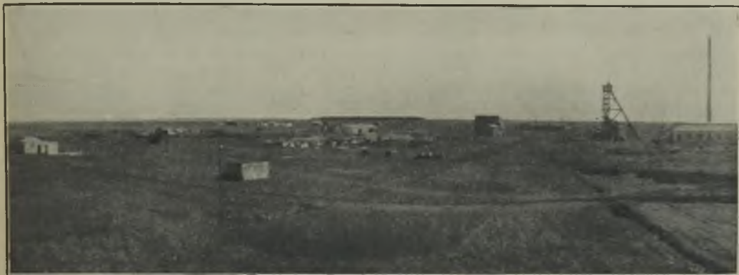
FIG. 4.—START OF EXCAVATION WORK: THE PLANT SITE IN APRIL, 1931.
