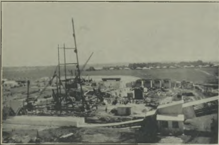
FIG. 6.—ERECTION OF HEADGEAR AT NO. 2 SHAFT.
